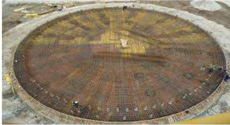
**Figure 4.2.** Plain slab type foundation <sup>[24]</sup>
