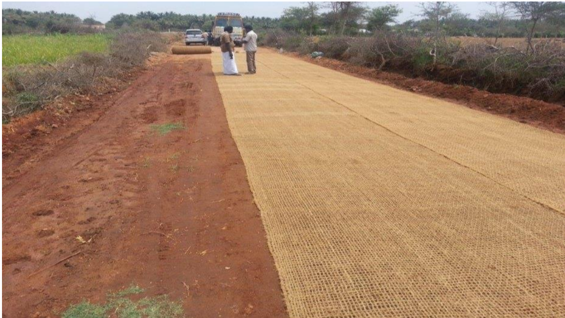
Figure 1.2: Use of Coir Geotextile for Road Construction
