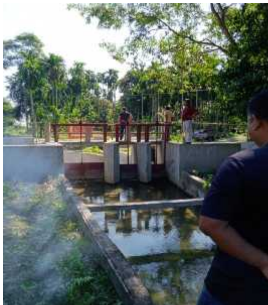
Fig 3.5 Cross regulator gates at the Junction point of main and branch canals
