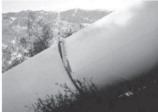
**Figure 3.5.** Locally buckled steel gas pipeline in the compression zone at North slope of Terminal Hill, 1994 Northridge earthquake (EERI, 1995)
