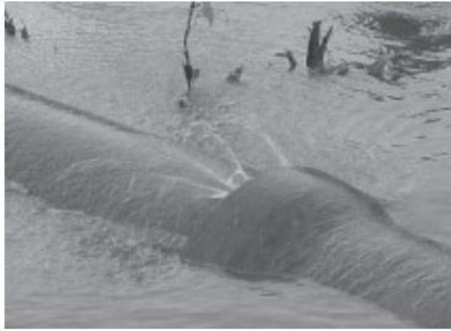
**Figure 3.10.** Water supply pipeline at Shippy Ghat, Port Blair, experienced a leak at the bell and spigot joint due to bending during the M9.0 Sumatra earthquake in 2004 (Photo: Suresh R Dash).
