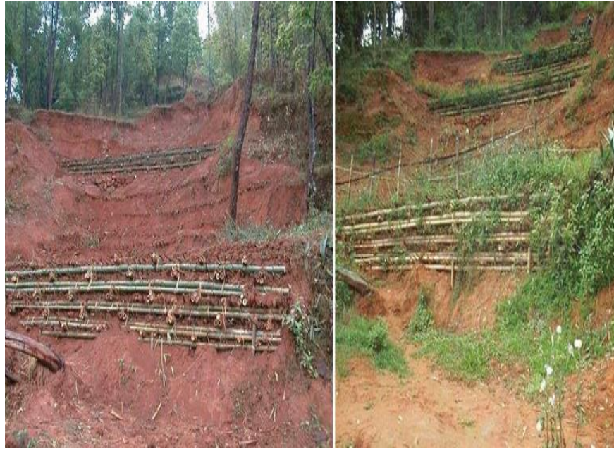
Fig 15: Bamboo stabilization of soil (source: www.intechopen.com )
