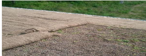
Fig14: Jute stabilization (source: www.pacificsoil.net )
