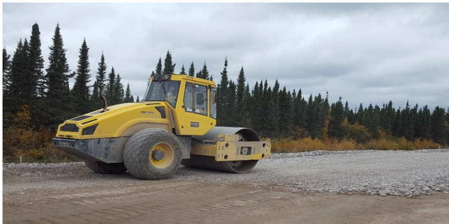
Fig 1: Static compaction being carried out. (sources: theconstructor.org)
