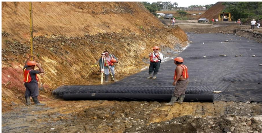
Fig 11: Geomembranes being used in road construction (source: industrialplastics.com.au )
