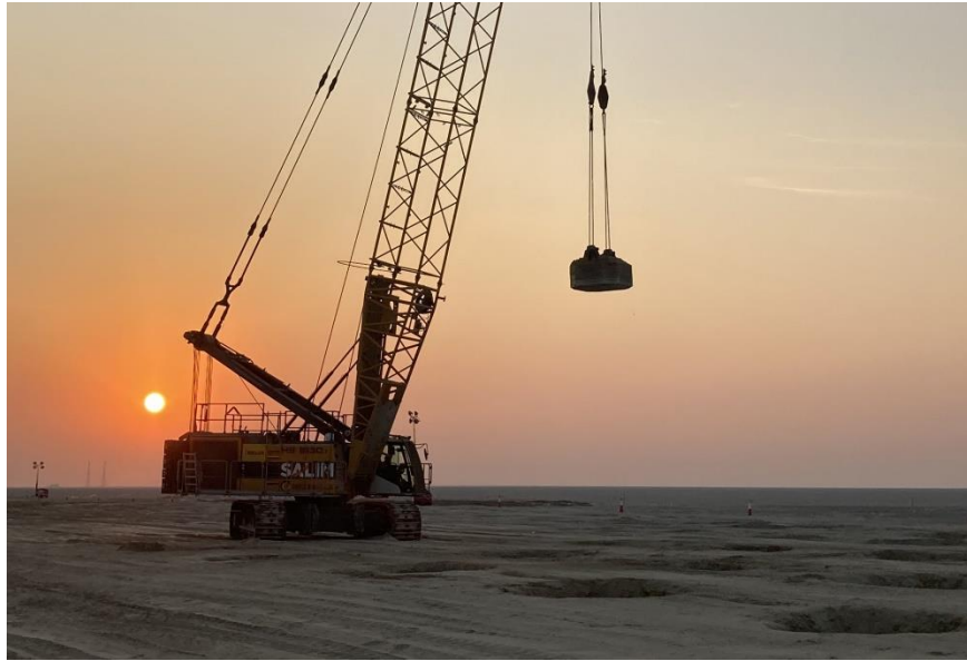
Fig 6: Dynamic compaction being carried out (sources: www.liebherr.com )
