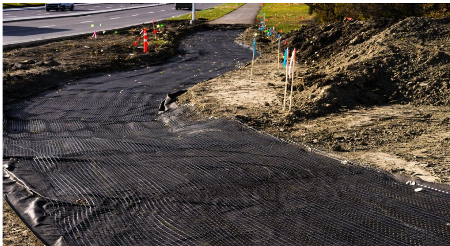
Fig 9: Geotextile membrane (sources: www.nyengineers.com )
