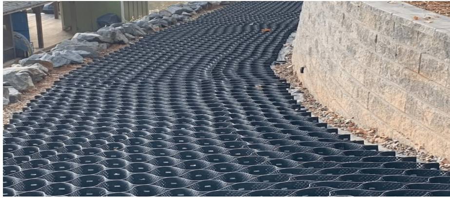
Fig 12: Geocells used to stabilise soil (source: geosyntheticsmagazine.com)
