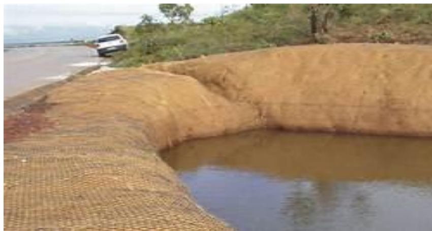
Fig 13: Coir stabilization near water bodies (source:gharpedia.com)
