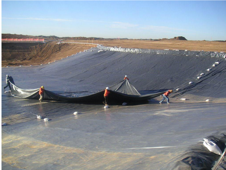
Figure 4.2: Synthetic Clay Liner
