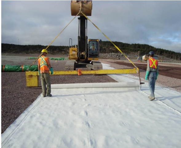
Fig 1.2: Installation of GCL
