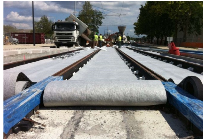
Fig 1.5: GCL on Road and Rail Construction
