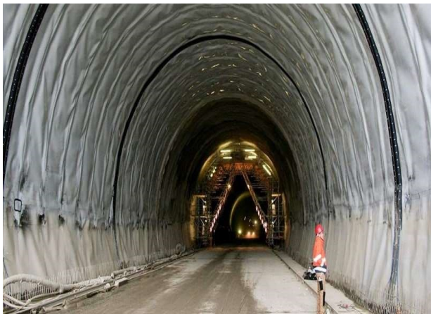
Fig 1.4: GCL on Tunnel Construction
