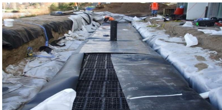
Fig 1.6: GCL Stormwater Management
