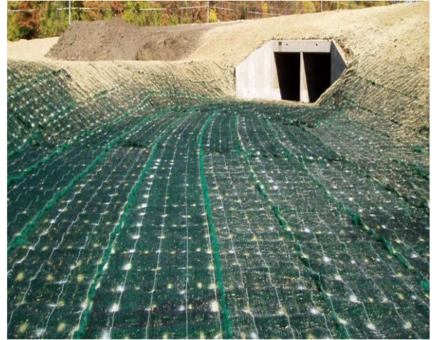
Fig 1.3: GCL for Slope Stability
