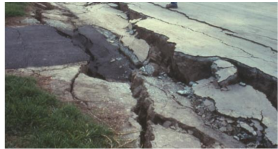
Fig 14: Lateral spread damage in California, USA
