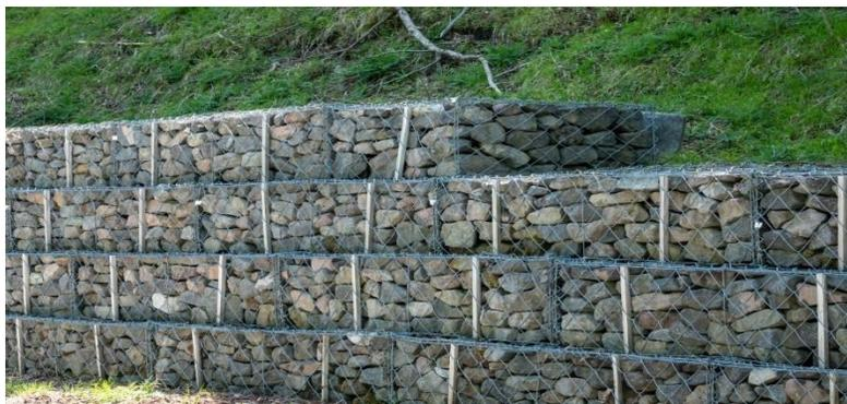
**Fig.1.5: Gabion Walls**
