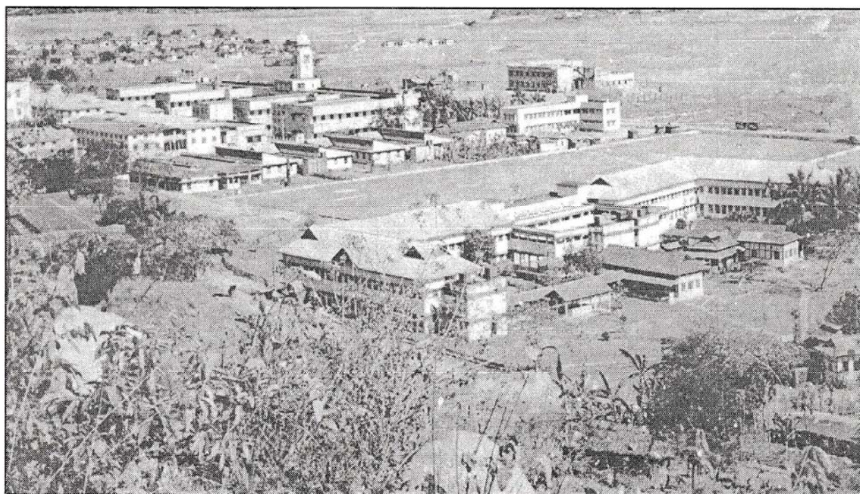
An overview of the college complex. Chemical Engineering building is also seen.
