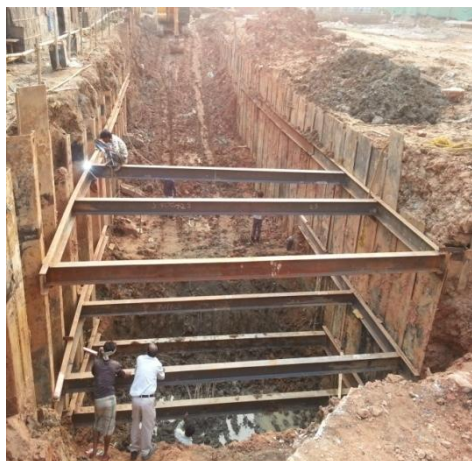
Plate 1a. Top-down excavation with cross-lot bracing
